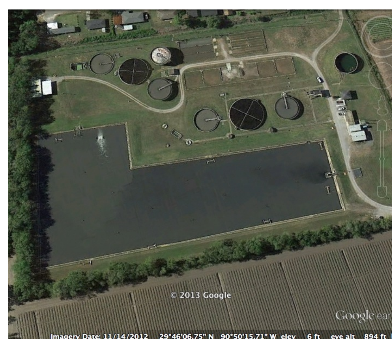
Figure 2. Thibodaux sewage treatment plant
